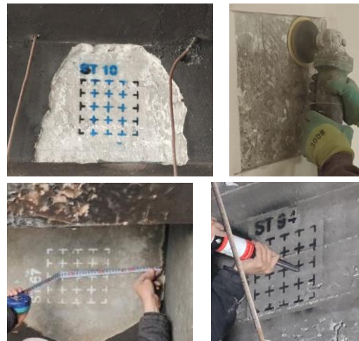
Fig. 6 Arrangements for hammer test at each station.
