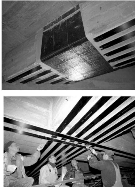
Fig. 1 Flexural and shear strengthening technique [14].
