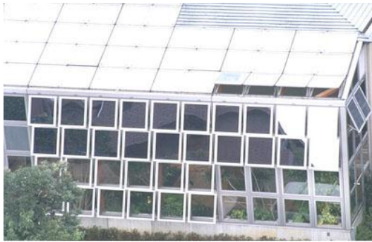
Back of the TRON Intelligent House
