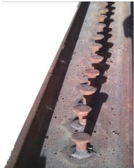
Plate1: The steel channel with its attached headed studs for beam TB –U45
