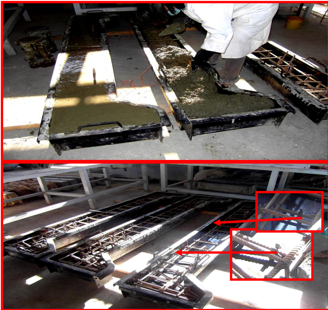
Figure (3) Columns Casting.
